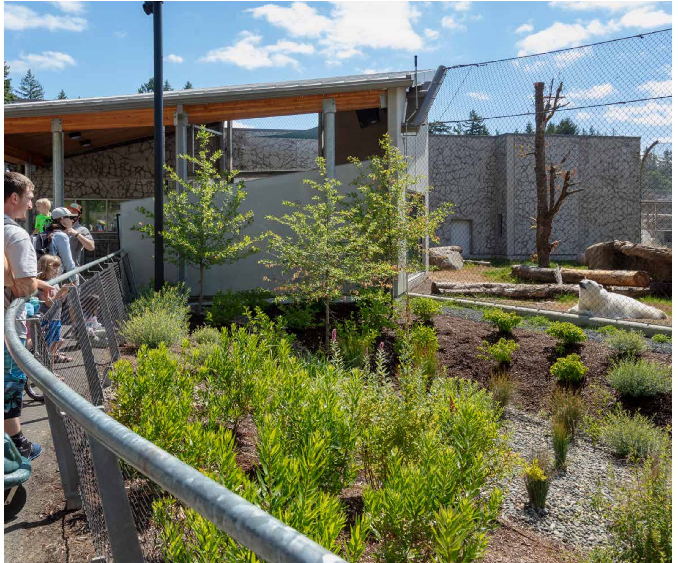
Green stormwater facility at Polar Passage
