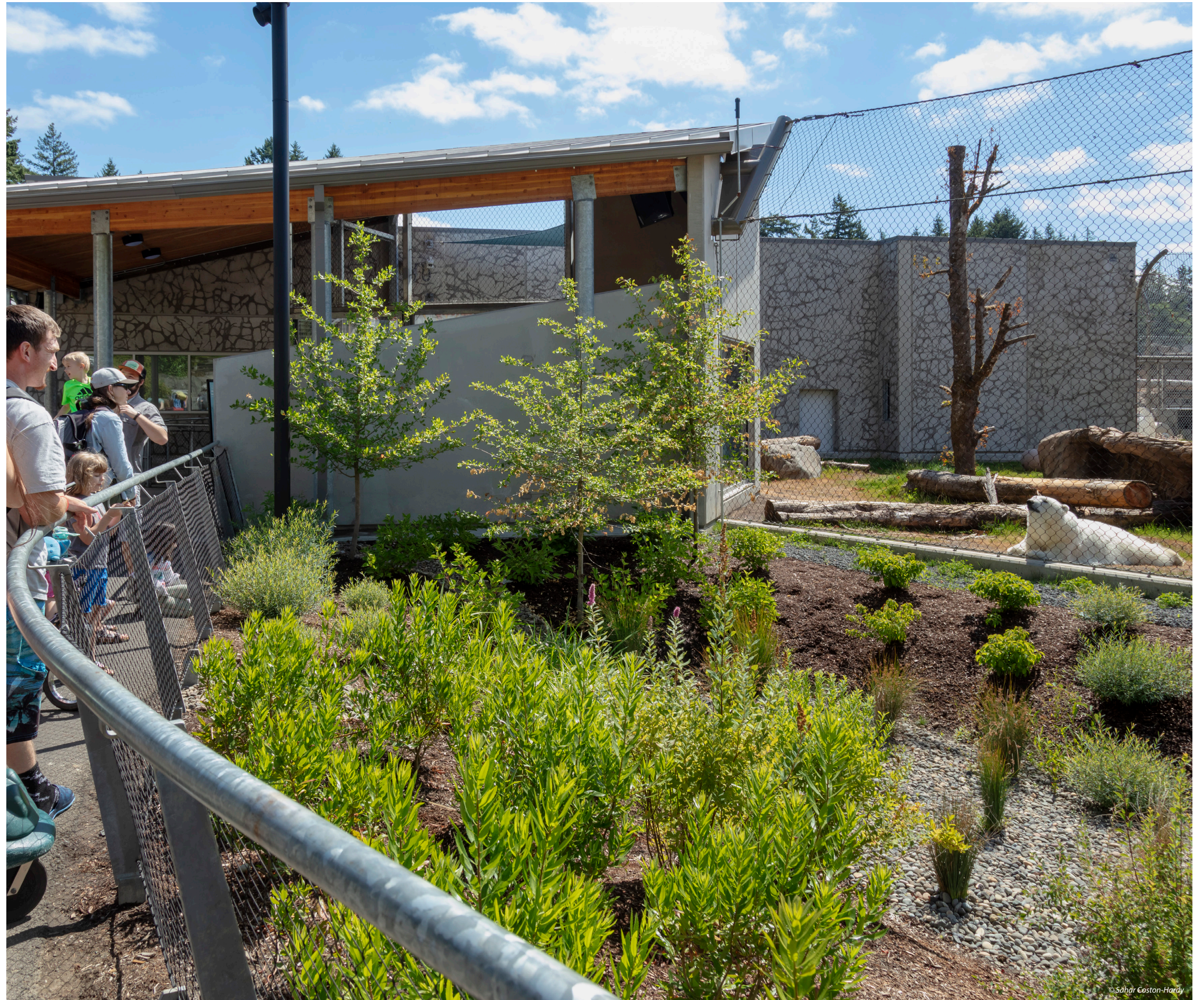
Green stormwater facility at Polar Passage
